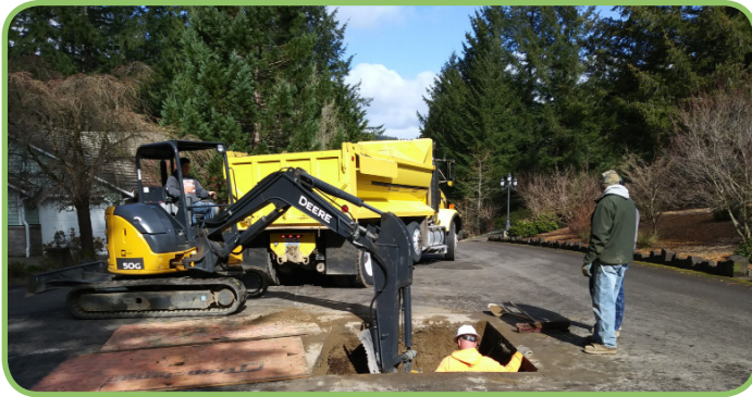
With the valve replacement project well under way, seven more distribution valves were replaced along Rocky Mountain Drive and McLane Creek Court.
