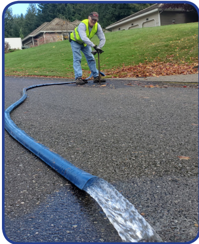
Pete Valenski flushes the water system twice a year to purge it from accumulated dirt and impurities.
