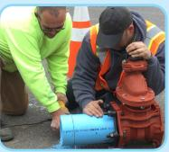
Measuring the precise length of the water pipe was important in order to get a correct fit. **Pete Valinske**, the Cougar Ridge Water Committee Chair, assists the crew and was present for the valve replacement installation.
