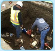
Once the holes were dug in the street, it was possible to see where the valves were located that were going to be replaced.
